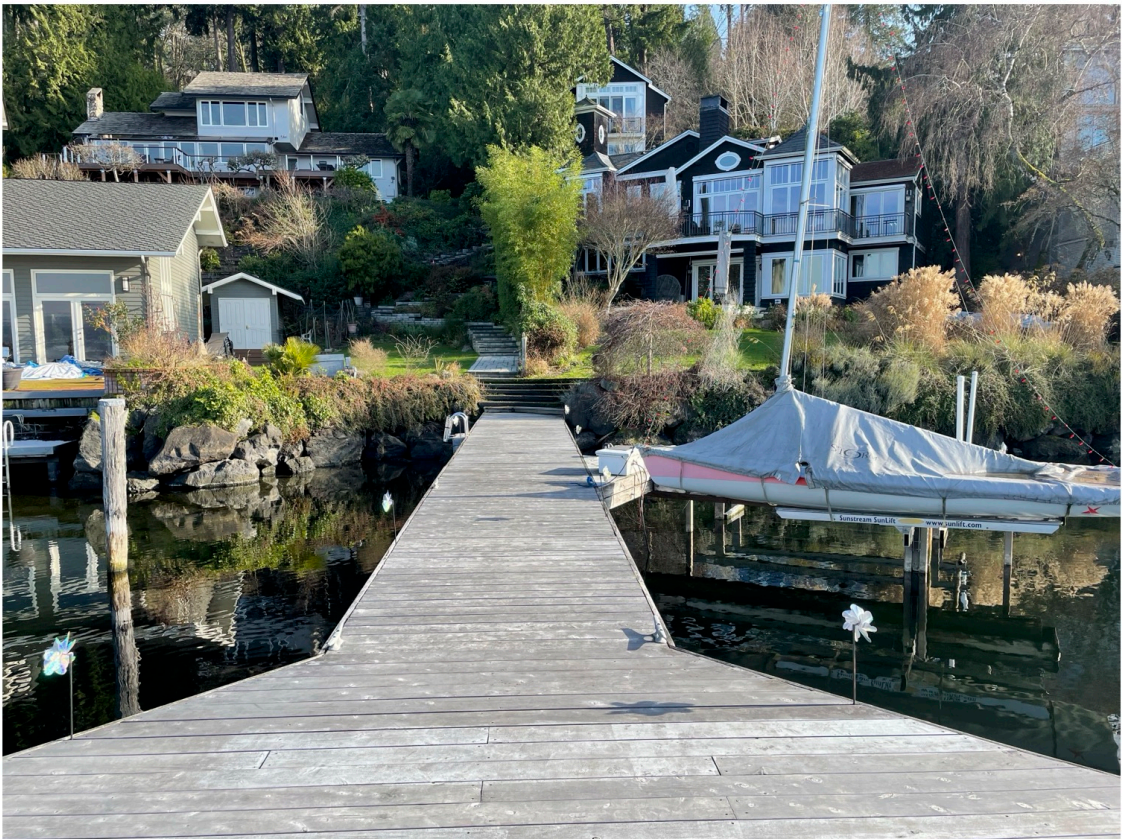
Photo 2 - Existing dock looking landward.
